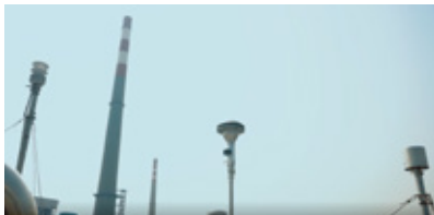
5G distributed point monitoring
