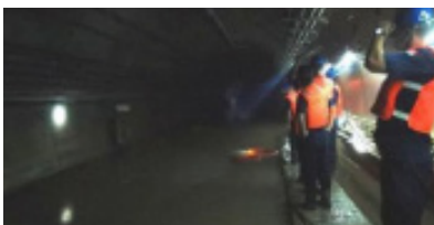
▲ Identification of track water logging
