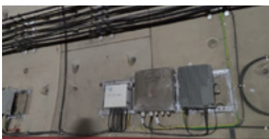
▲ anomaly monitoring of tunnel wall box
