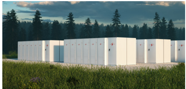
Lithium-ion battery storage
