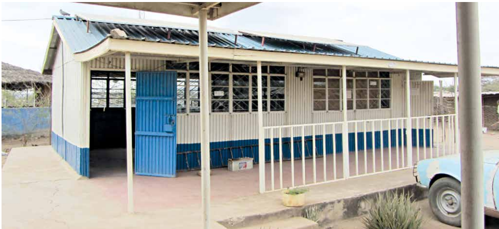
Existing but inoperative energy centre
